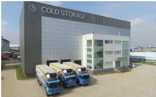
Gambar 2. 1 Cold Storage Statis (Sumber: Foto KKP)
